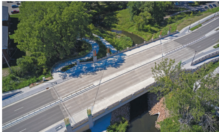
UPGRADE Kimley-Horn provided design services for the reconstruction of Louisiana Avenue over Minnehaha Creek in St. Louis County in Minnesota.
