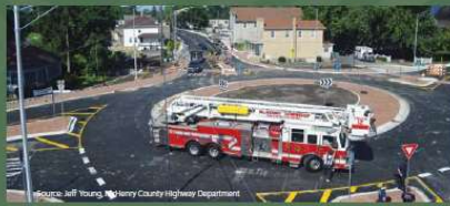
Source: Jeff Young, Henry County Highway Department
