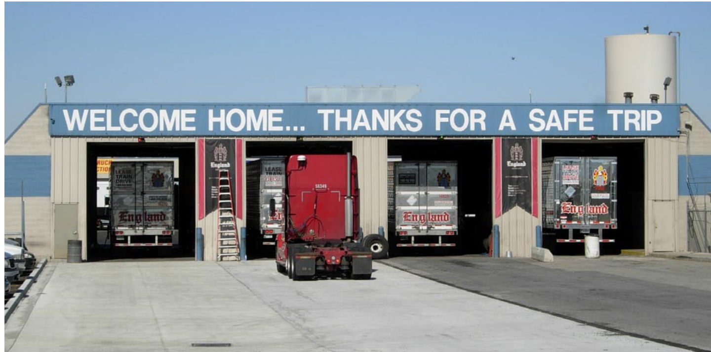
Truck servicing facility at C.R. England headquarters in Salt Lake City.
